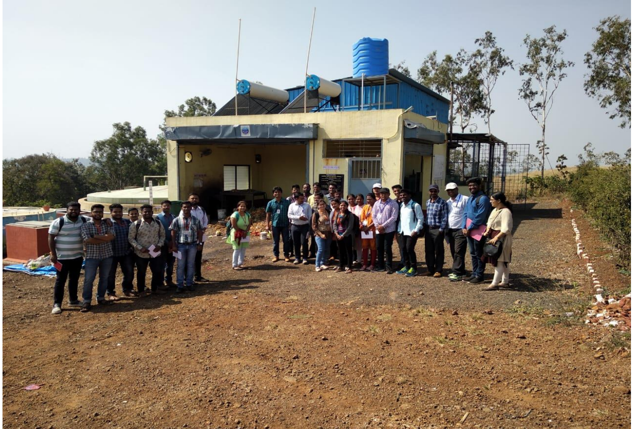
FOOD WASTE TREATMENT PLANT, KOLHAPUR
